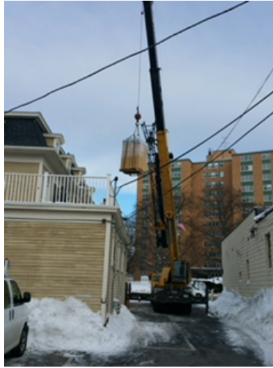
At left, Replacing Jeremiahs Inn heating system.
